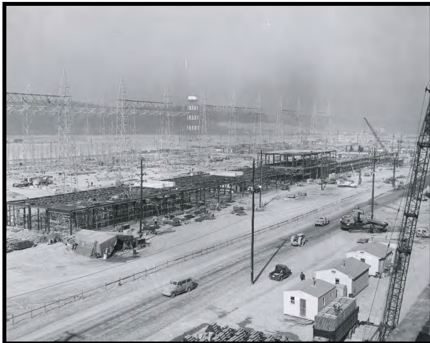
Figure 22: Steel Framework for the X-530 Electrical Switchyard Complex, November 1953
