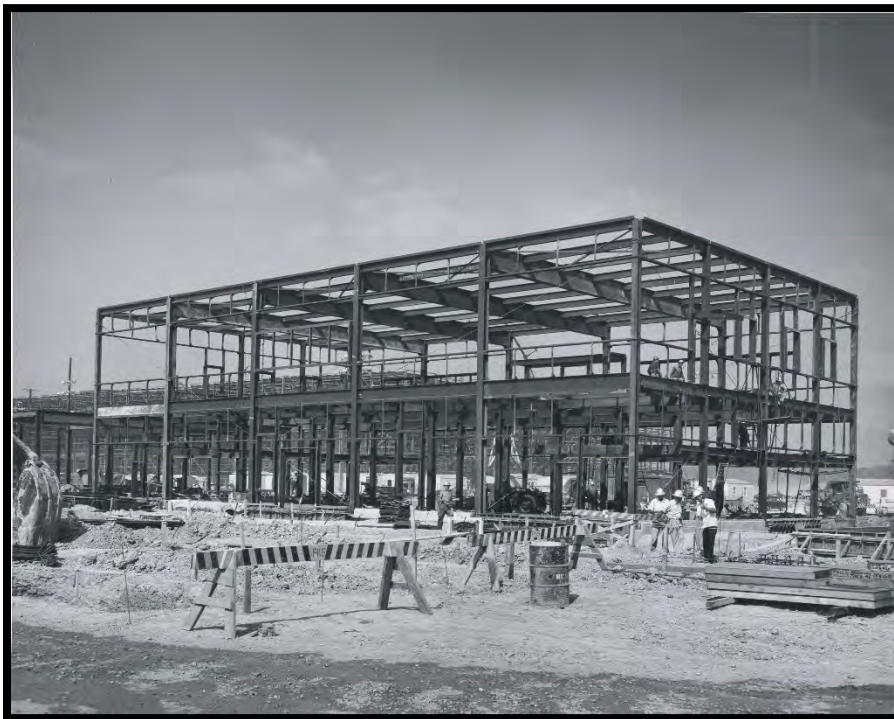
Figure 21: Steel Framework for the X-530 Electrical Switchyard Complex, October 1953
