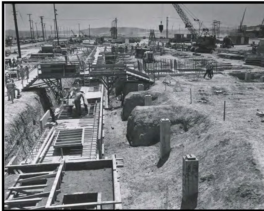
Figure 16: Foundation Work for the X-530 Electrical Switchyard Complex, September 1953
