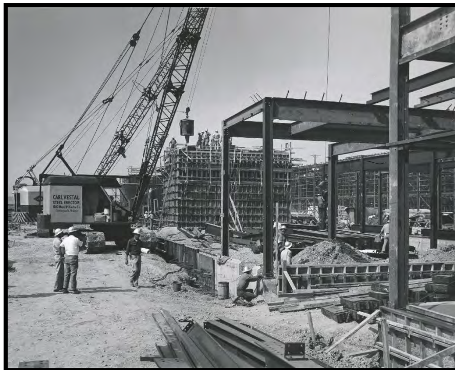
Figure 19: Foundation Work for the X-530 Electrical Switchyard Complex, September 1953
