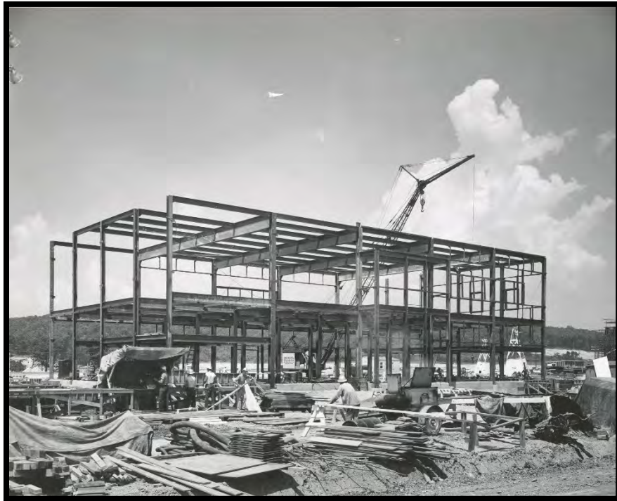
Figure 20: Steel Framework for the X-530 Electrical Switchyard Complex, October 1953
