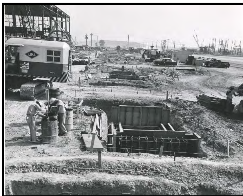
Figure 15: Grading and Foundation Work for the X-530 Electrical Switchyard Complex, August 1953
