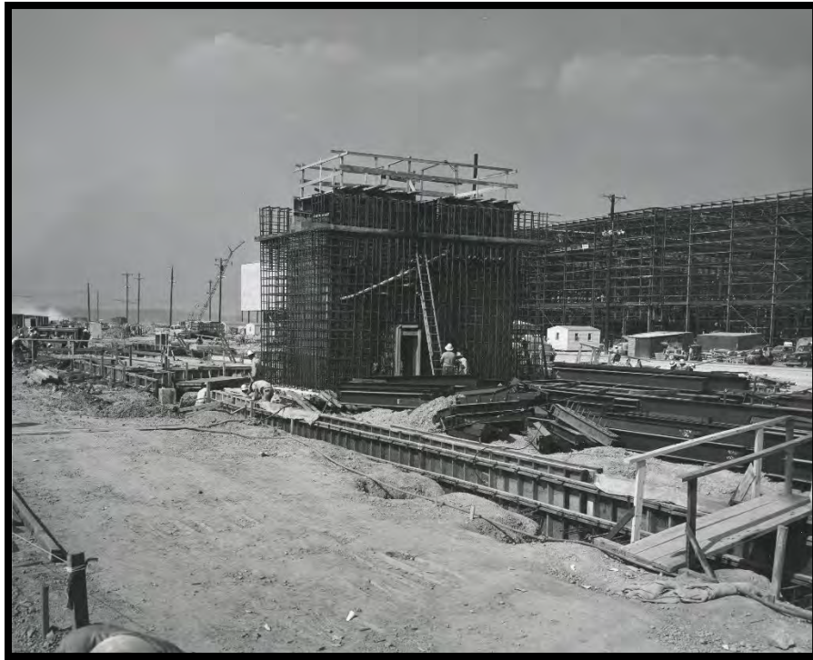
Figure 18: Foundation Work for the X-530 Electrical Switchyard Complex, September 1953
