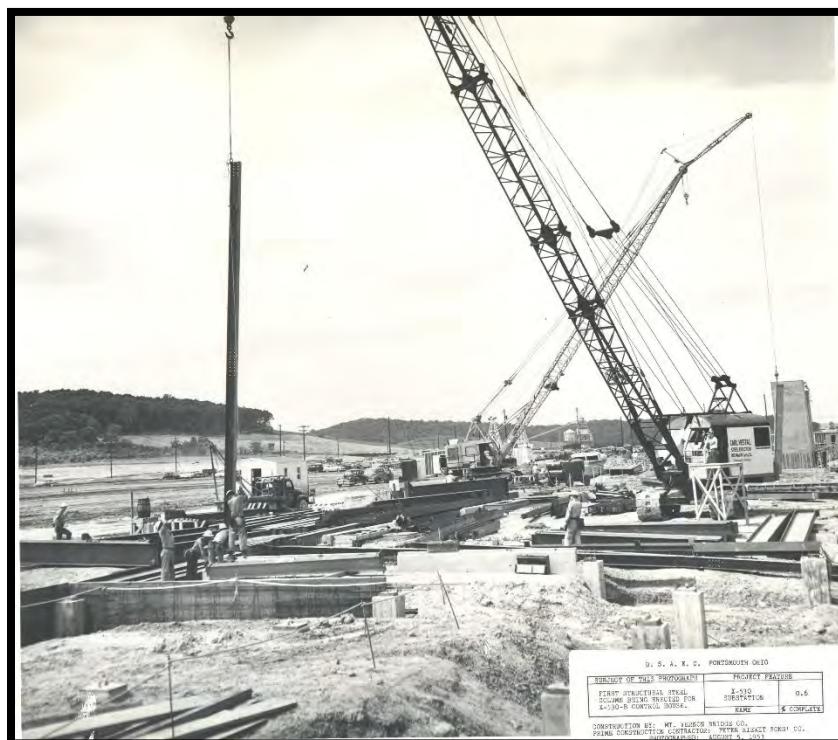
Figure 14: First Structural Steel Column Being Erected for the X-530B Switch House, August 1953
