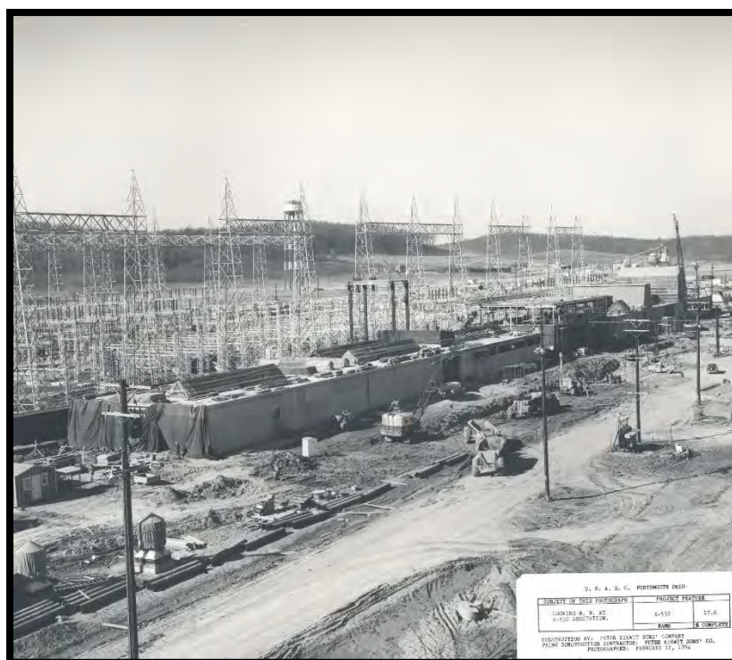
Figure 24: Steel Framework for the X-530 Electrical Switchyard Complex, December 1953
