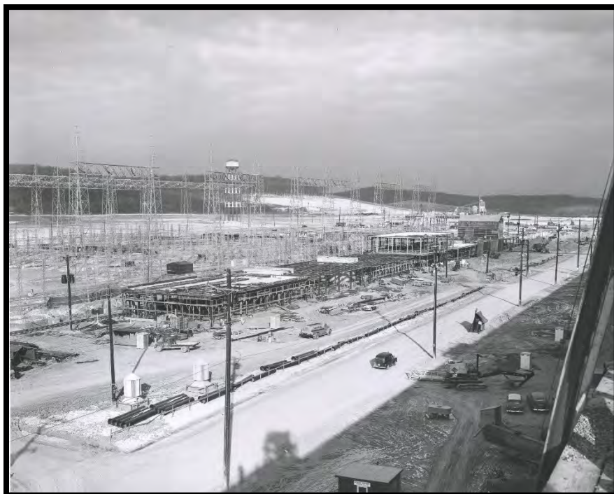
Figure 23: Steel Framework for the X-530 Electrical Switchyard Complex, December 1953
