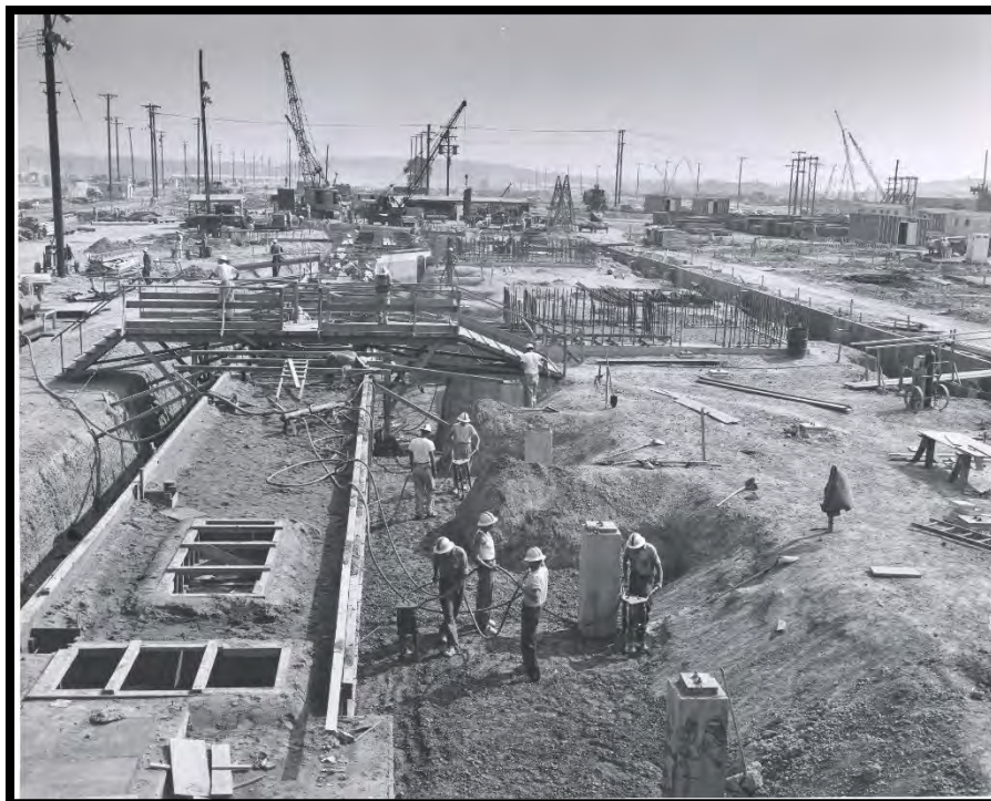
Figure 17: Foundation Work for the X-530 Electrical Switchyard Complex, September 1953
